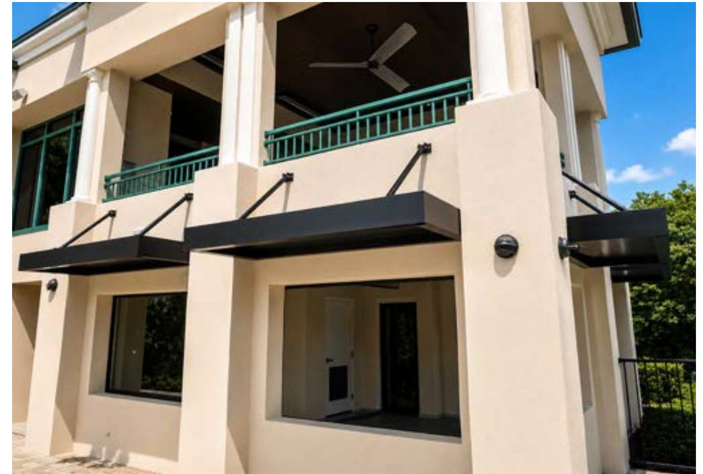
The Vinoy Golf Course, St. Petersburg Decking Canopy
